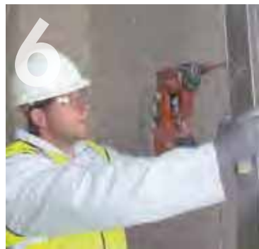
6 Fixing Knauf Deep Flange 'U' Channel to studs at door opening.
