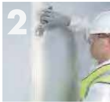
Bedding Knauf Joint Tape.
