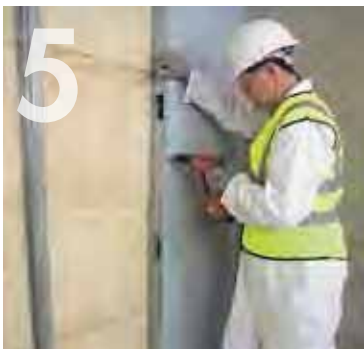
5 Fixing Knauf Plasterboard to the Knauf 'C' Studs.
