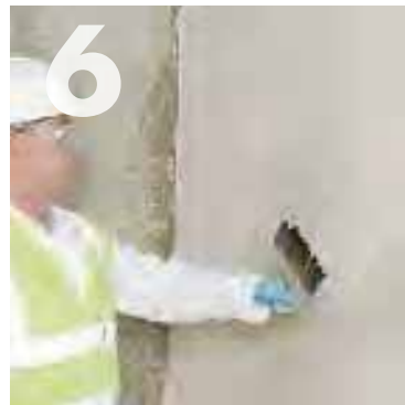
Flicking the water over the surface prior to using the sponge float.
