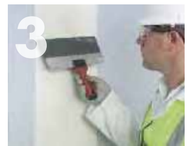
Applying first coat of Knauf Joint Cement Easy Sand.
