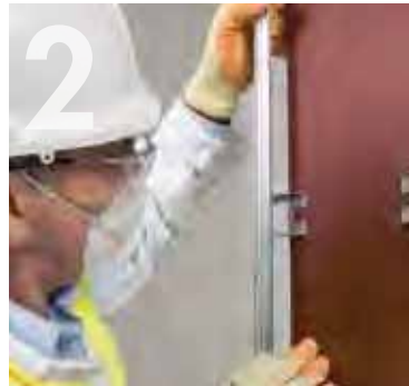
Pushing Knauf 'C' Channel into the Knauf Fixing Clips.
