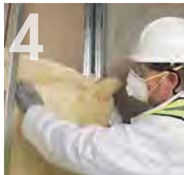
4 Inserting Knauf insulation quilt between the Knauf 'C' Studs.
