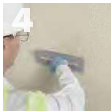
4 Trowel Knauf MPFinish flat as it is applied.
