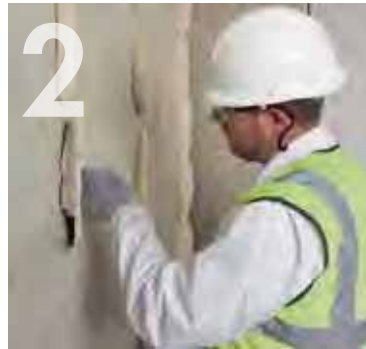
Applying Knauf Plasterboard Adhesive dabs at the required centres.
