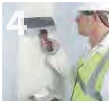
Applying the first coat of Knauf Joint Cement Easy Sand.
