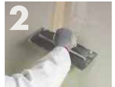
Apply Knauf Joint Filler over the tape.
