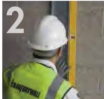
Fixing Knauf 'U' Channel to form the perimeter frame.
