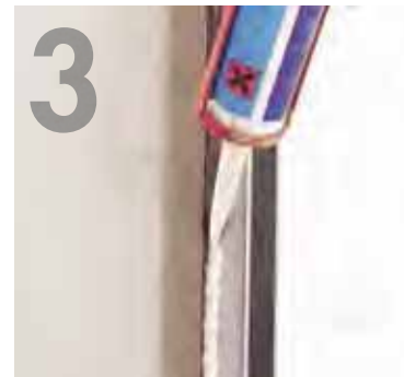
Applying Knauf Aquapanel Interior Joint Adhesive
