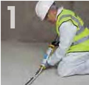
1 Applying continuous beads of Knauf Sealant to perimeter framing.
