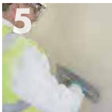
5 Apply the first dry trowel once the plaster has picked up.
