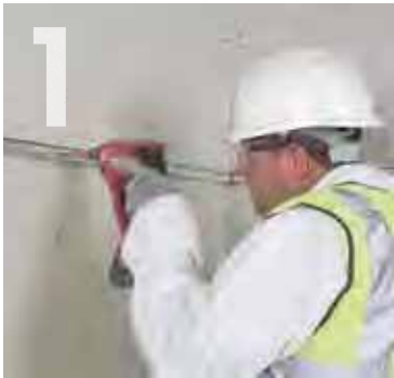
Fixing Knauf MF Perimeter Channel.
