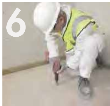
6 Screwing the sheets of Brio together using the correct size Knauf Brio Screws.
