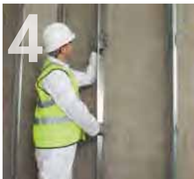
Adjusting the stud position.
