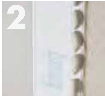
Ensure all holes are completely filled.
