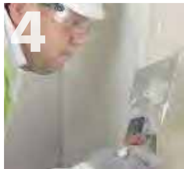
Apply second coat to 175mm each side of the corner.
