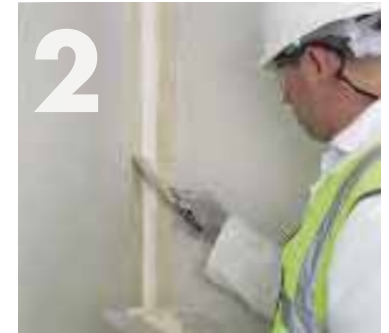
Bedding Knauf Joint Tape.
