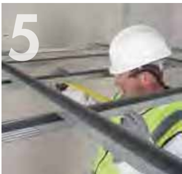
Measuring the distance between lower Knauf 'C' Channels.
