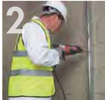
2 Fixing the first stud to the adjoining wall.
