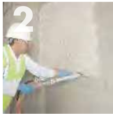
Spray Knauf MP75 in overlapping bands.
