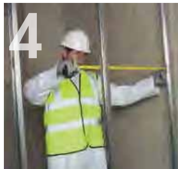
4 Positioning studs at 900mm centres.
