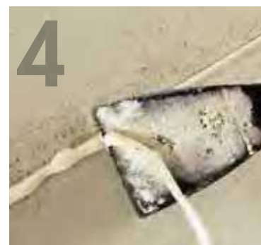
Scraping off the excess adhesive once cured
