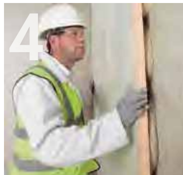
Offering up Knauf Thermal Laminate for a better thermal performance.
