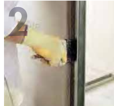
Cleaning the edges with a wet brush
