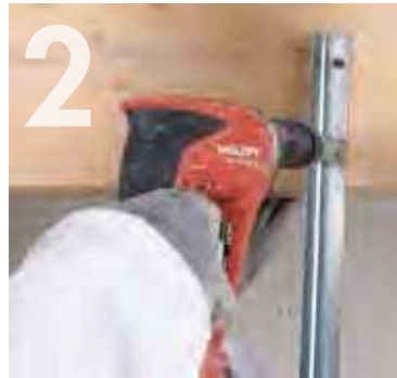
Fixing the Knauf Angle Section to joist to form hanger.
