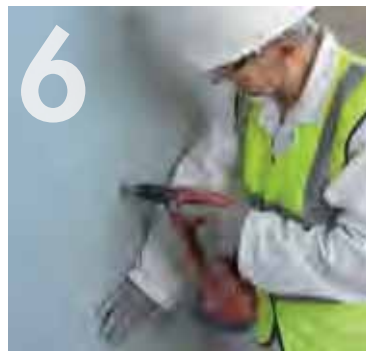
Fixing Knauf Soundshield to the frame.
