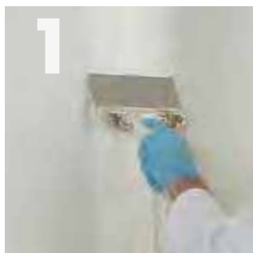
1 Filling the joints.
