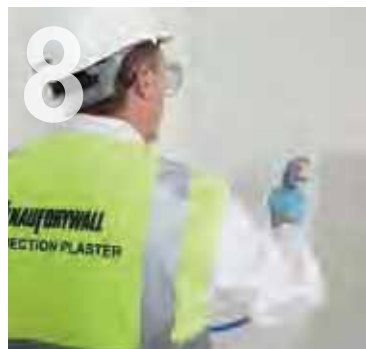
Finishing using Knauf plaster.
