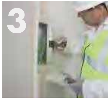
Applying the first layer of Knauf Joint Filler.
