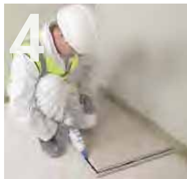
4 Applying Knauf Brio Joint Adhesive to the edge of the sheet.
