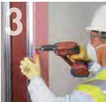
Fixing Knauf Fireshield onto the Knauf 'C' Channels.
