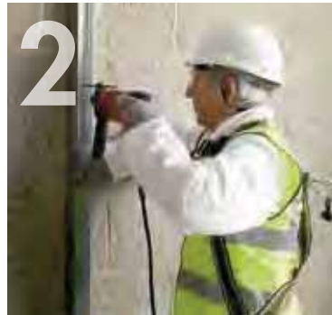
Fixing Knauf 'J' Channel to the abutting wall.
