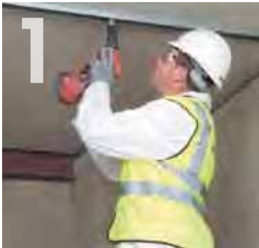
1 Fixing the head track.
