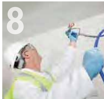
Spray applied Knauf Readymix Plasters make finishing ceilings safe, easy and fast.
