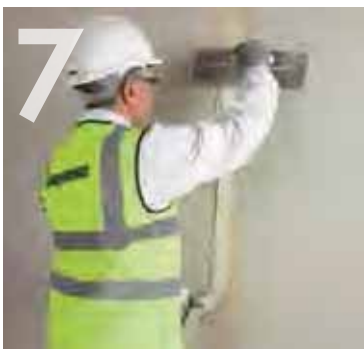
Taping and jointing for a seamless finish.
