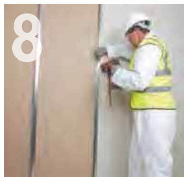
8 Fixing Knauf Plasterboard to the completed framework.
