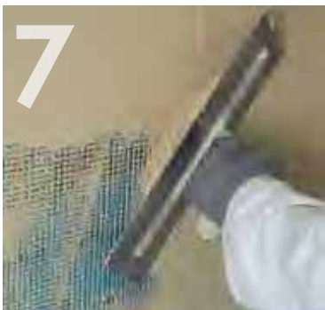
Covering mesh with basecoat.
