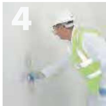
Levelling Knauf Airless flat using a spatula.
