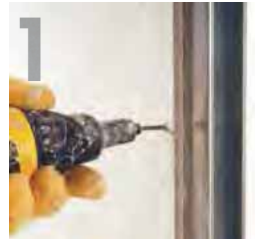
Fixing Knauf Aquapanel Interior cement board
