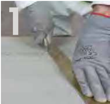
Scoring Knauf Aquapanel Exterior with a knife.
