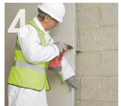
Fixing Knauf Plasterboard to the Knauf 'C' Channel.
