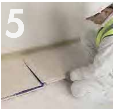
5 Laying the second sheet of Knauf Brio.
