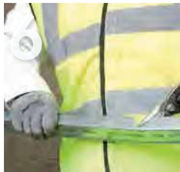
6 Snip and bend Knauf 'U' Channel to form door head.
