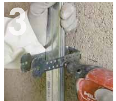
Fixing Knauf 'C' Channel to the Knauf Universal Bracket.
