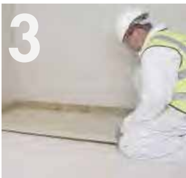
3 Laying the first sheet of Knauf Brio.
