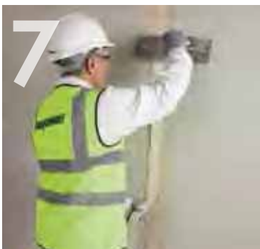
7 Taping and jointing for a seamless finish.
