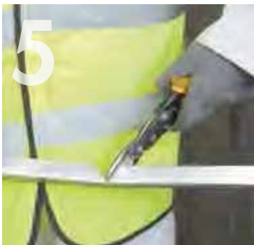
5 Snip and bend back Knauf Deep Flange 'U' Channel to form the door frame.
