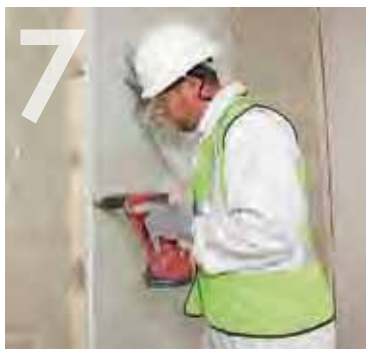
Fixing Knauf Plasterboard onto the Knauf MF Channel.
