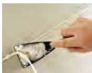
Scraping off the excess adhesive once dry.
