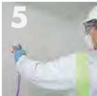
Applying the second coat of Knauf Airless.
