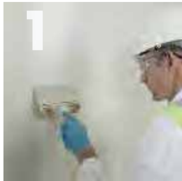
Filling the joints.
