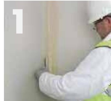
Ensure the joint is completely filled.
