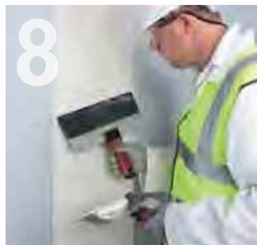
8 Tape and joint for a seamless finish.
