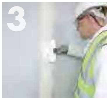
Applying Knauf Joint Cement Easy Sand over the tape.
