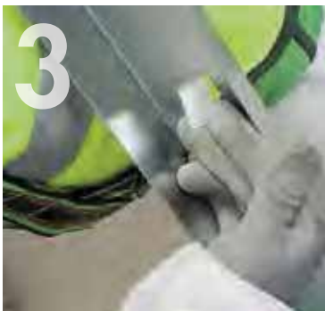
The retention clips are easy to release with the Knauf Core Board in place.
