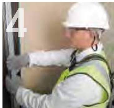
Positioning Knauf C-T Stud to lock Knauf Core Board into place.
