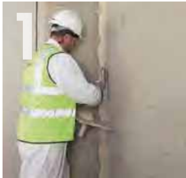
Applying a continuous band of Knauf Plasterboard Adhesive around the perimeter.
