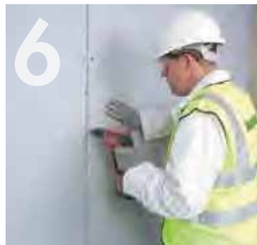
6 Stagger the boards, to ensure all joints overlap.
