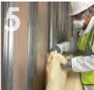
Installing insulation quilt horizontally between the studs.
