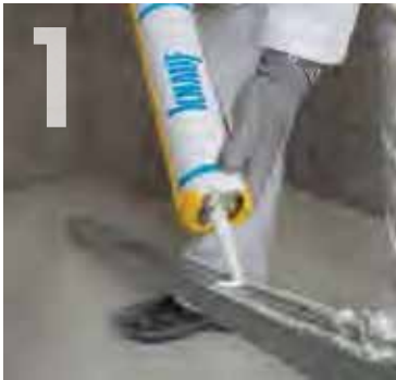
Applying two continuous beads of Knauf Sealant to perimeter framing.
