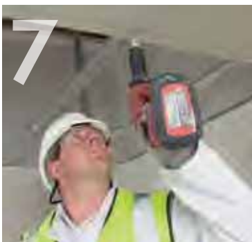
Screw fixing the Knauf Plasterboard to the lower Knauf 'C' Channels.
