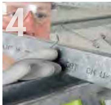
Connect the Knauf Primary Support Channel to the Knauf MF Ceiling Channel with Knauf MF Connecting Clips.
