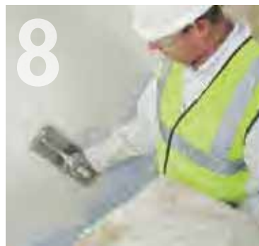
8 Finishing using Knauf plaster.
