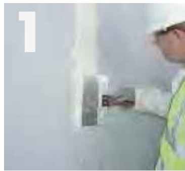
Applying Knauf Joint Cement Easy Sand.
