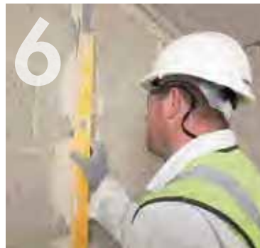
Ensuring Knauf MF Channels are fixed plumb.
