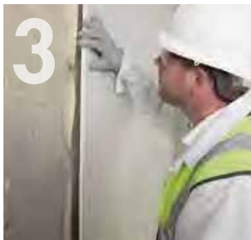
Offering up Knauf Plasterboard and pressing into place.
