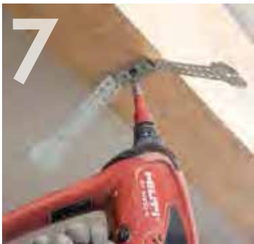
Knauf Universal Brackets can be used as an alternative to Knauf Angle Section for shallow voids.
