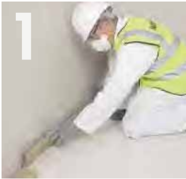
1 Installing Knauf Brio Edge Strip to the room perimeter.
