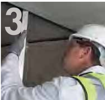
3 Twisting Knauf Acoustic 'C' Studs into position.
