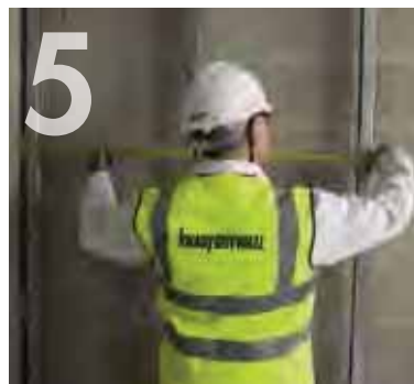
Measuring the distance between studs.
