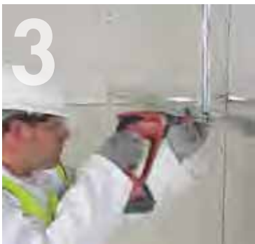
Fixing the Knauf Angle Section to Knauf MF Primary Support Channel.
