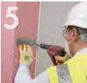
Fixing Knauf Flat Fixing Plate between layers.
