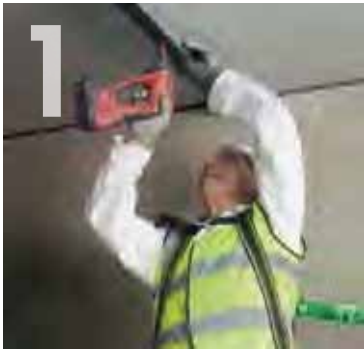
Fixing Knauf 'J' Channel to the soffit.
