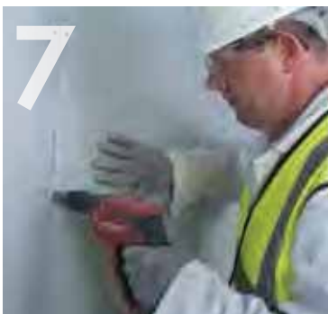
7 Fixing the 15mm Knauf Soundshield to the Knauf Acoustic 'C' Stud.
