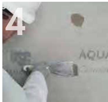
Covering screw heads with Knauf Aquapanel Joint Filler - Grey.
