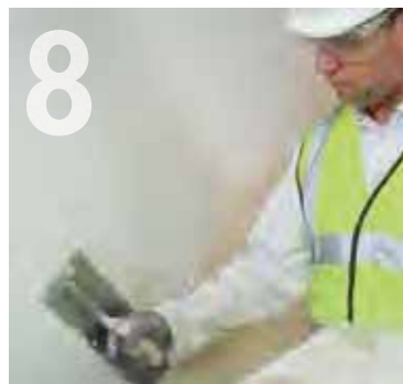
Finishing using Knauf Plaster.
