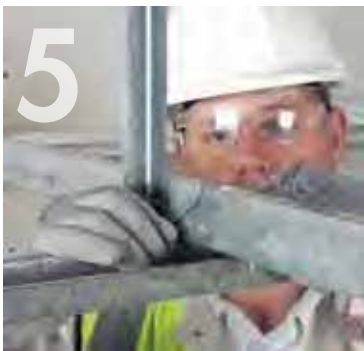
Adjusting the Knauf MF Ceiling Channel.
