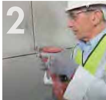
Fixing the boards to the background members.
