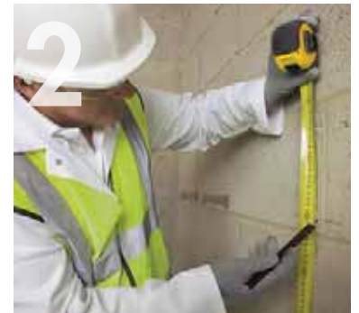
Marking position for the Knauf Universal Bracket.
