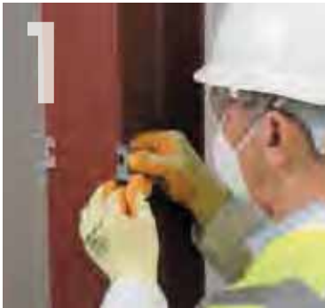
Installing Knauf Fixing Clips.
