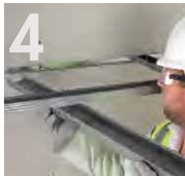
Positioning lower Knauf 'C' Channel into Knauf Perimeter Channel.
