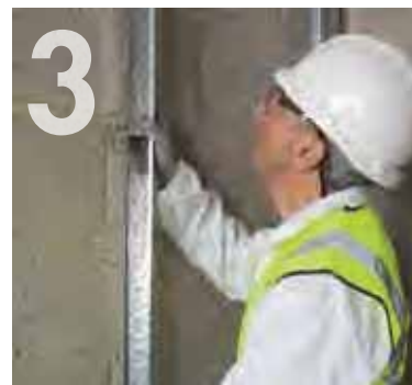
Twisting Knauf 'I' Studs into place.
