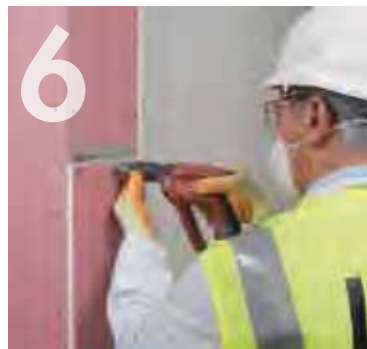
Fixing outer layer of Knauf Fireshield.
