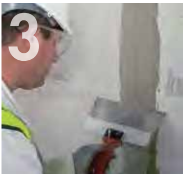
Embedding Knauf Aquapanel Exterior Joint Tape.
