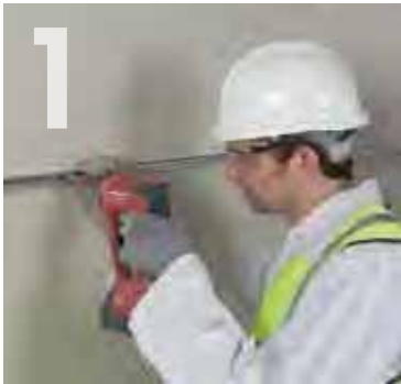
Fixing Knauf Perimeter Channel.
