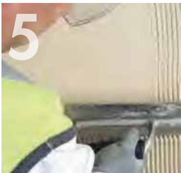
Applying notches within the basecoat.
