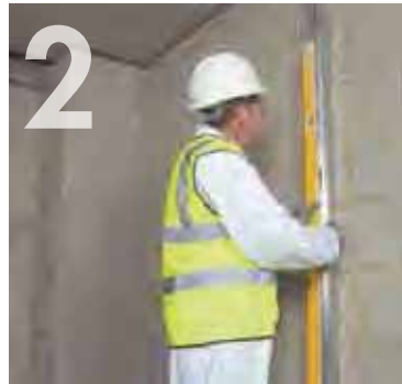
2 Fixing Knauf 'C' Stud to form the partition frame abutment.
