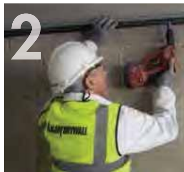
Installing head track.
