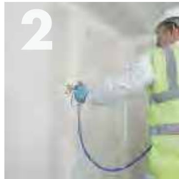
Applying the first coat of Knauf Airless.
