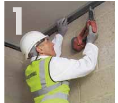
Fixing Knauf 'U' Channel - Perimeter Support to the soffit.
