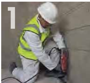
Installing floor track.
