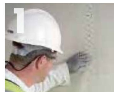
Apply self adhesive Knauf Fibre Tape to joint.
