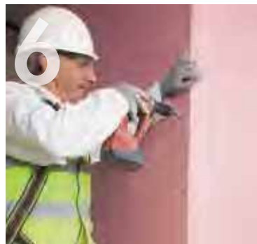
Fixing Knauf Fireshield.
