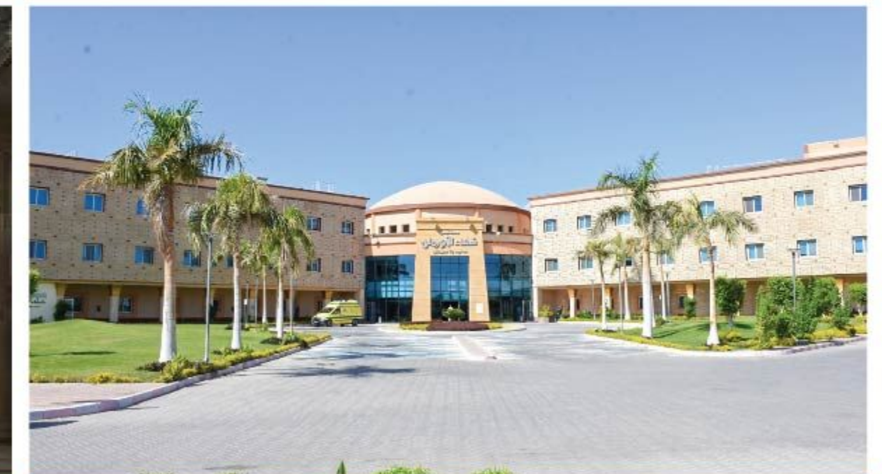
Projects in Luxor and Aswan: Shifa Orman Hospital in Luxor. More than 300 units for health insurance.
